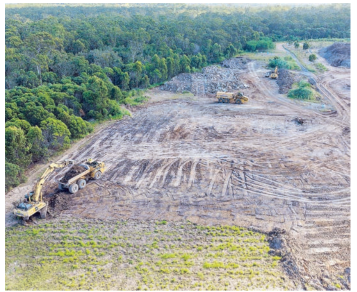
The Gateway Stage 4 works underway.
