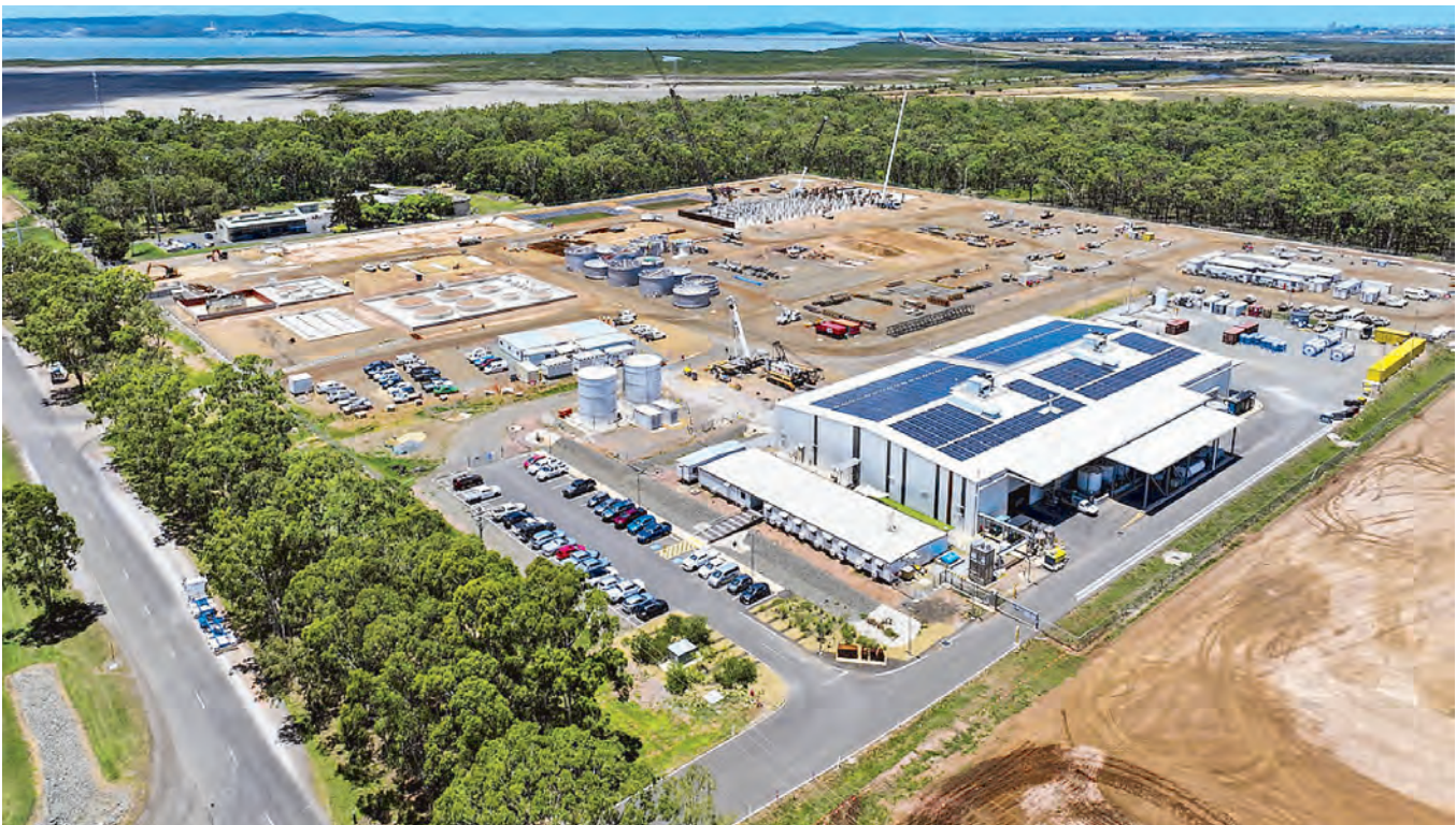
An aerial view of stage two works at the Alpha HPA site in Gladstone this month. (Supplied)
