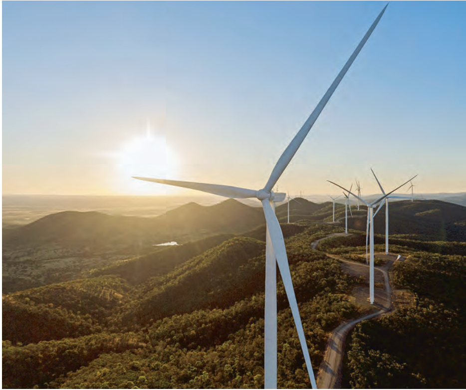
Clarke Creek Wind Farm has confirmed the presence of asbestos in the brake pads of lifts used to access the top of the Clarke Creek Wind Farm's 207m-tall turbines. (Supplied)
