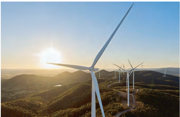
Spanning 100 turbines, Clarke Creek Wind Farms is the biggest wind farm opened in Australia this year. (Supplied)
