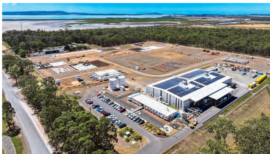
the $30 million investment by the Queensland Investment Corporation will advance construction of Alpha HPA's Stage Two HPA First Project in Gladstone. (Alpha HPA)
