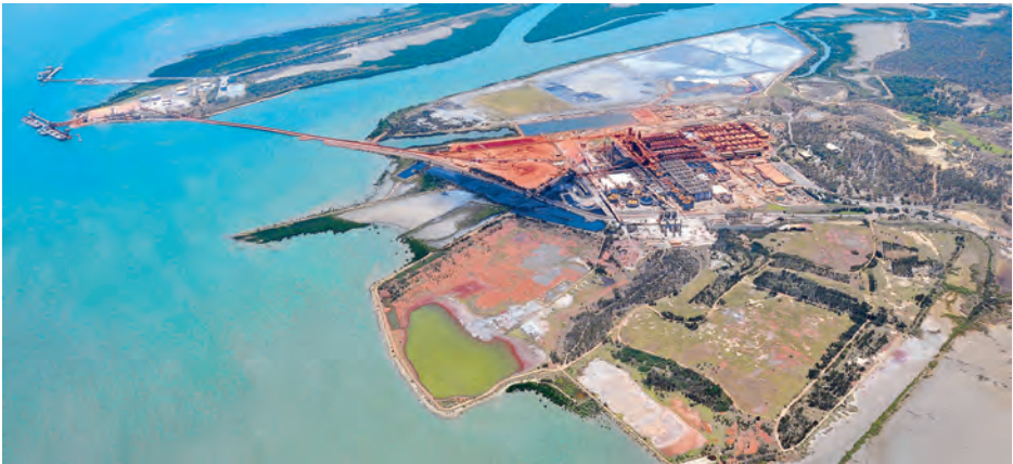
Part of the industrial landscape for 58 years, QAL was fined $1 million in a Gladstone court on Monday, 22 September, for environmental breaches relating to the rupture of a high-pressure pipe bearing sodium hydroxide on 22 March, 2022. (Supplied)
