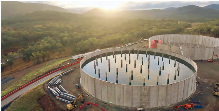
Water has begun flowing into the Aldoga Reservoirs for the first time, marking a major construction milestone in the $983 million Fitzroy to Gladstone Pipeline. (Supplied)
