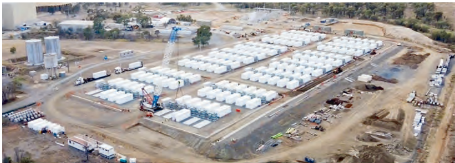
Each of the 324 Megapacks have been transported by truck from the Port of Brisbane and installed at the Stanwell site.
