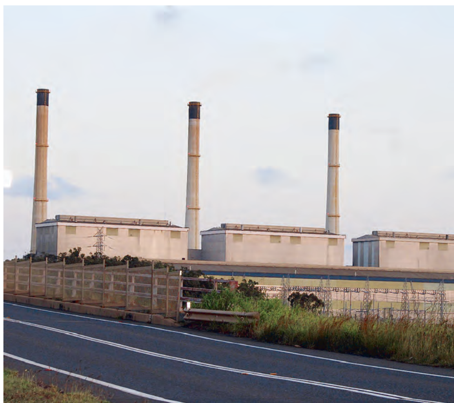
The Gladstone Power Station.
