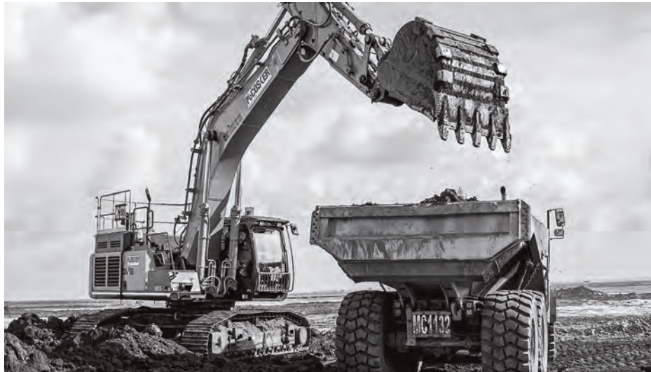
An excavator load at Gove in the Northern Territory.
