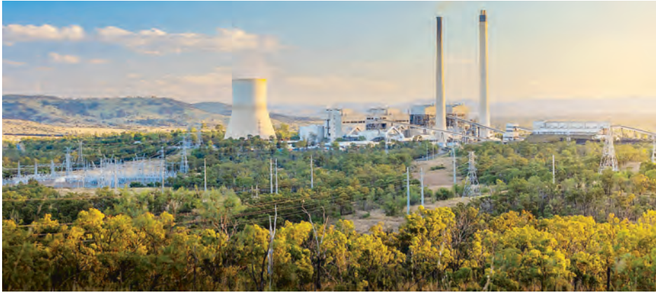
CS Energy has released a damning report into the 4 April explosion at Callide Power Station. The station's embattled C3 Unit is undergoing an $80 million overhaul. (Supplied)
