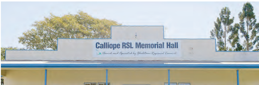
The Calliope RSL Memorial Hall will be repurposed into a central and accessible community space including five consulting rooms, two multi-purpose rooms, a meeting room and connection lounge.
