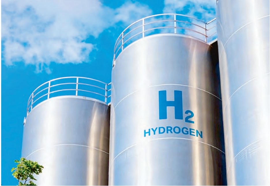
Stanwell has announced it has pulled out of the CQ-H2 project. (Stanwell.com)
