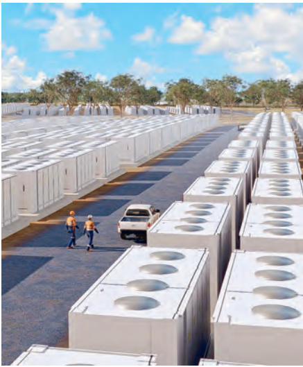
A Battery Energy Storage System proposed to be sited near the Lilyvale substation BESS is expected to have a storage capacity of 1600-2000MWh based on current technology. (Supplied)
