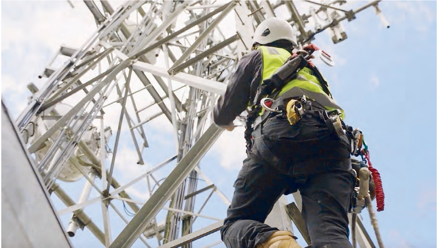
A series of Telstra upgrades and new construction projects are being rolled out across Central and Western Queensland over the next 12 months. (Telstra)
