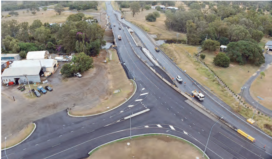
The Rockhampton Ring Road project had a hit a major milestone, with the first of 18 bridges completed.
