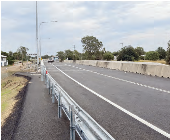
The new Lion Creek Bridge is open to traffic.
