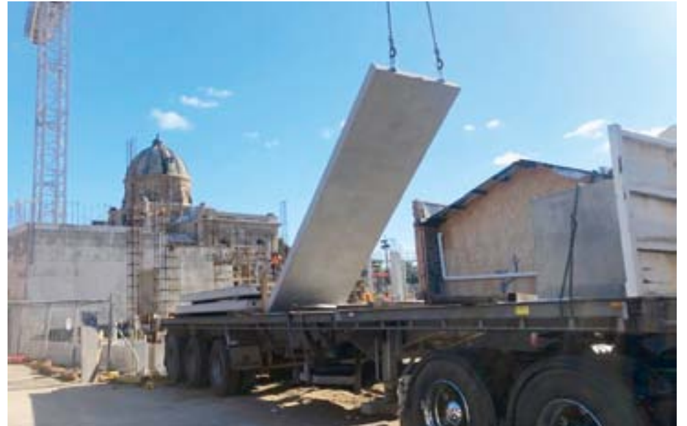
Wall panel erection at the Rockhampton Art Gallery.
