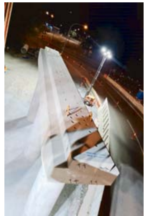
70T Headstock installed on the Smithfield Project (Cairns) for Albem Contractors.
