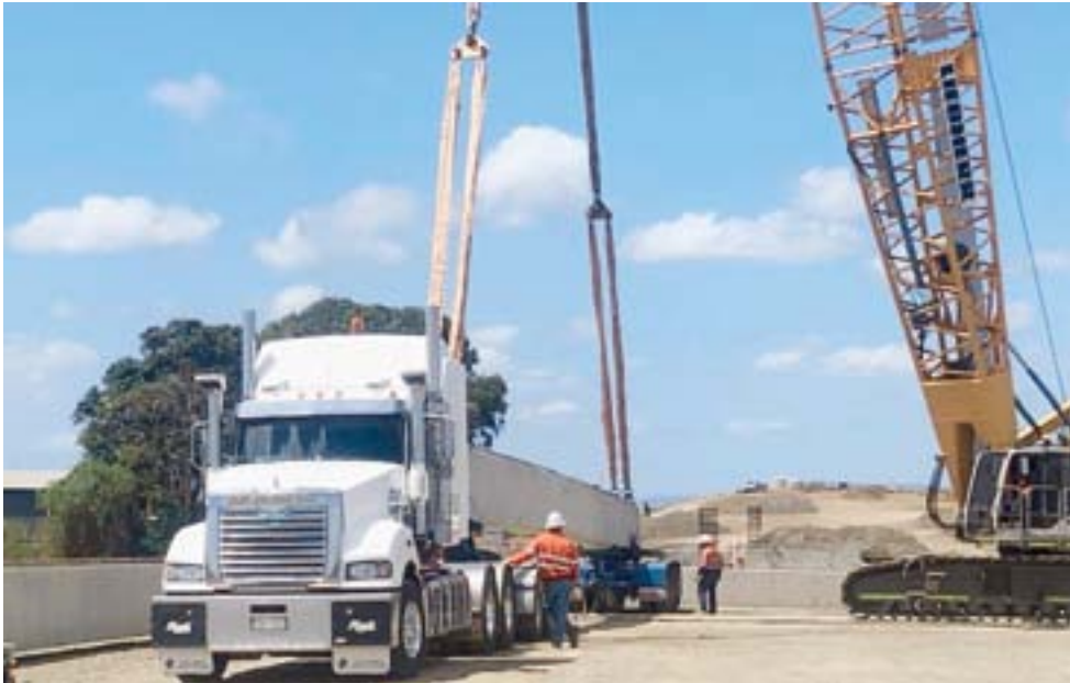
Bridge Decks being unloaded on Mackay Ring Road Project.
