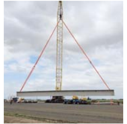
80T T-Girder unloading at Mackay Ring Road Project.
