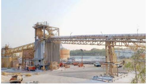
QAL replaced an alumina conveyor with a sealed airslide, eliminating airborne alumina during transfer.
